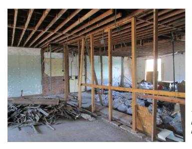
Third floor framing showing removed bearing wall and shoring repairs..
