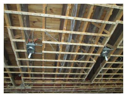
Third floor framing showing original framing members, repaired subfloor above, and secondary ceiling framing with some new electrical rough-ins.
