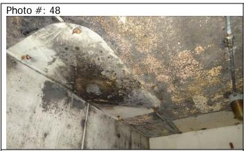
**Description:** View of mold in one of the walk-in refrigerator/freezers in the kitchen area.
