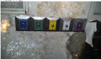
**Description:** View of ports on the wall indicating the use of various gases in this room. This room was likely used as an operating room. Eight of these rooms were observed in the basement.
