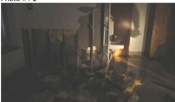
**Description:** View of room off main entrance. Sheetrock is damaged and insulation has been pulled from the wall. Standing pool of water in background is several inches deep.
