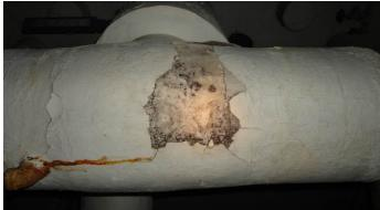
**Description:** View of pipe wrapping. Pipe wrapping appeared to be disturbed in many locations. Fibers could be seen as part of the wrapping material.
