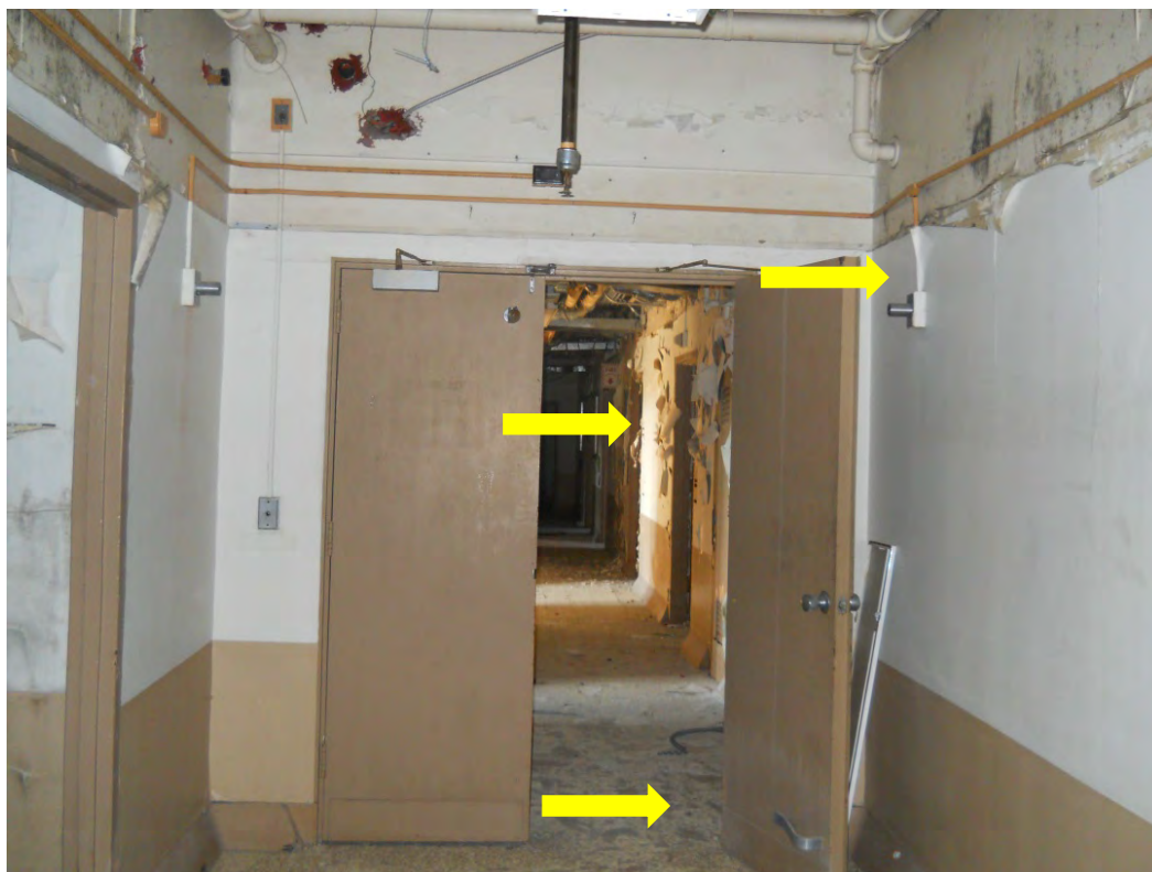
Photo 2 – Deteriorated wall finishings and flooring throughout hallway
