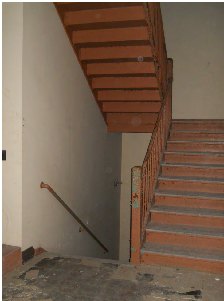
Photo 3 – Typical Stairwell with deteriorated painted surfaces and floor tile
