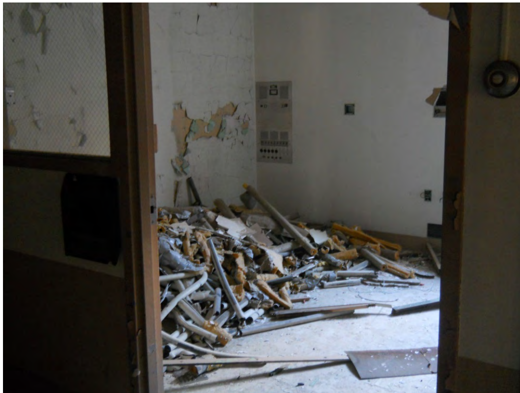
Photo 1 – Debris pile of various types of pipe insulation
