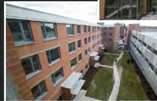
Pedestrian Access to Transit Center
