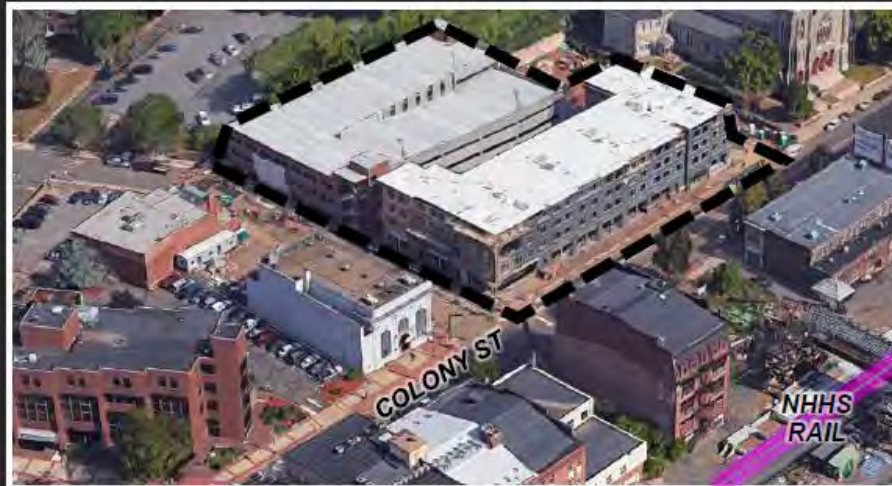
Mixed-Use Development – Construction Completed in 2016
