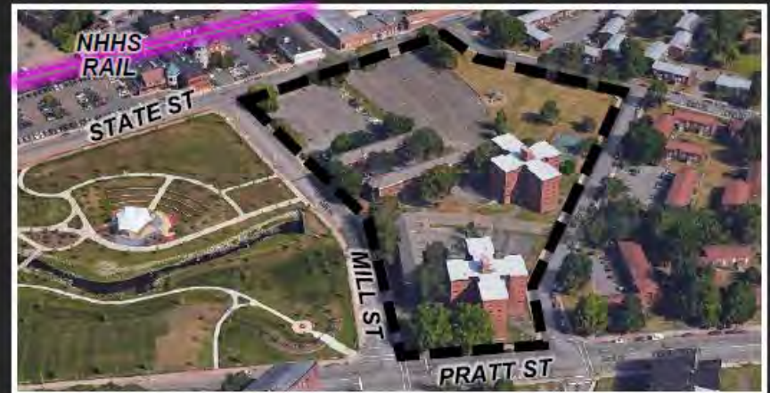
Current Mills Housing Complex and adjacent to New Meriden Green
