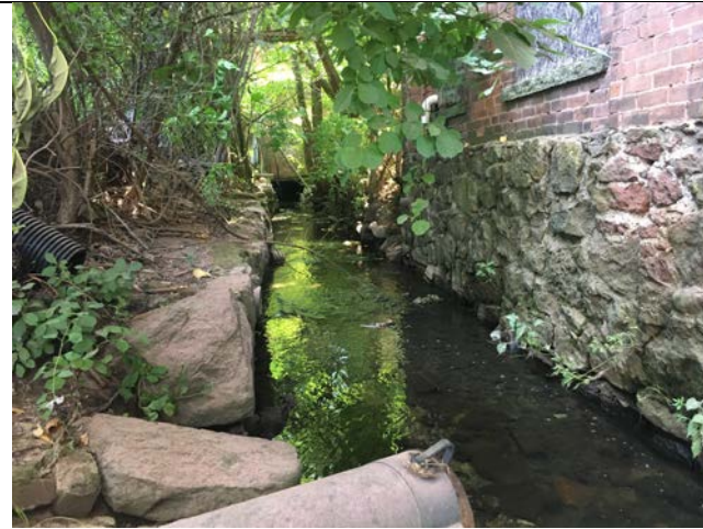
Clark Brook, facing south from the northern part of the brook. The pipe in the foreground was previously associated with site wastewater discharge.
